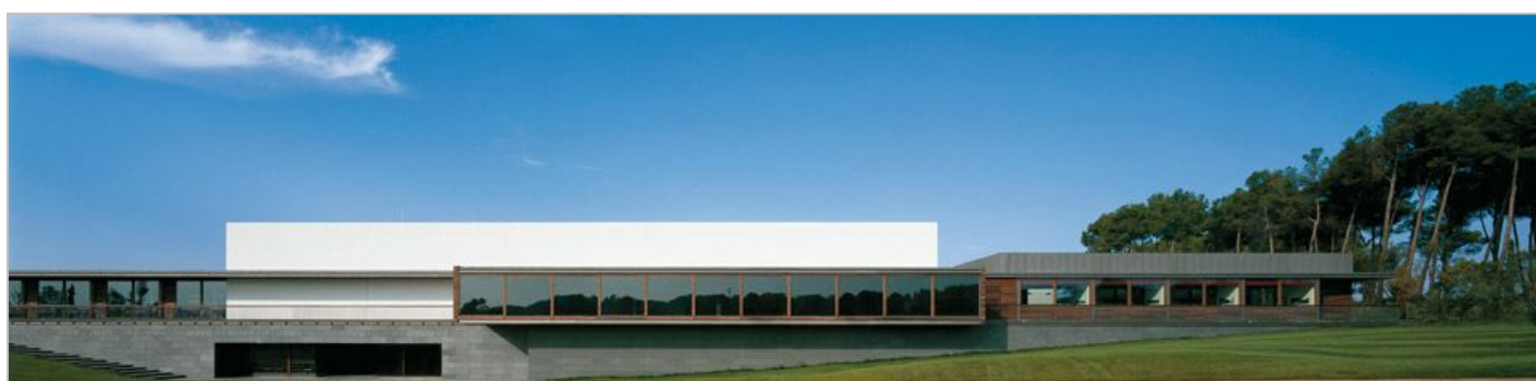
Club House – General view
