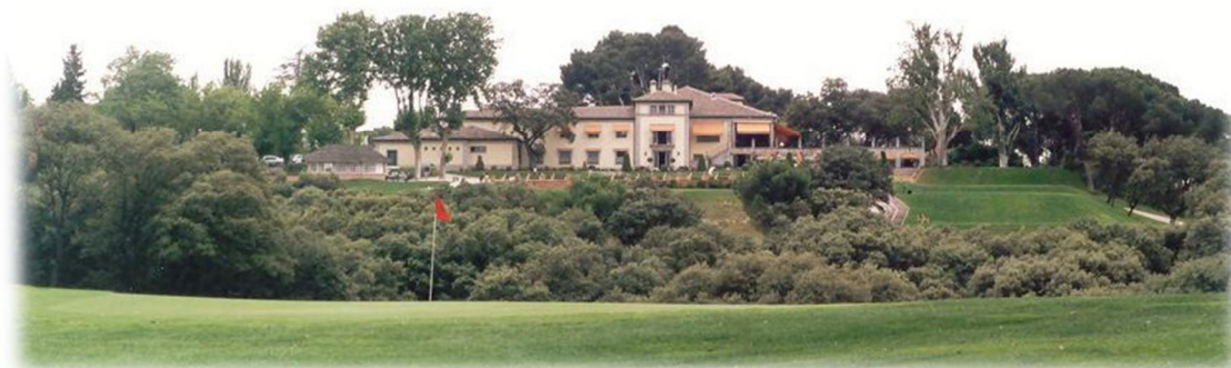
Club house general view
