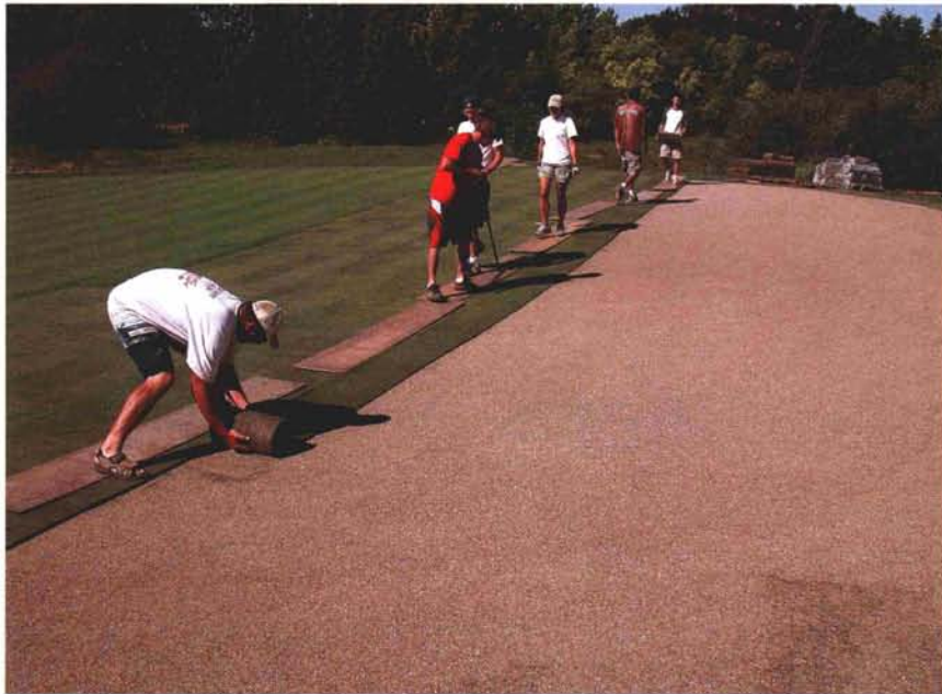
Using plywood helps to limit wear injury to sod and is a good tip during successful installation.
