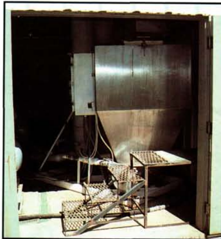
Acid injection and sulfur burners can be used to treat water with excess bicarbonate levels. Acidifying irrigation water to a pH of 6.5 reduces bicarbonates by approximately 50%.
