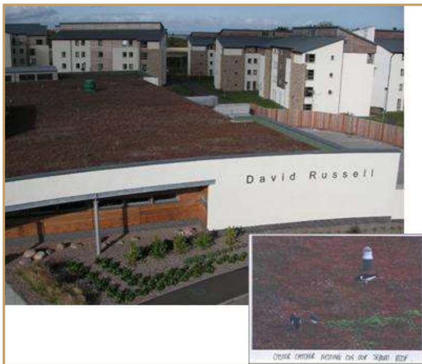
Green Roof at DRA
